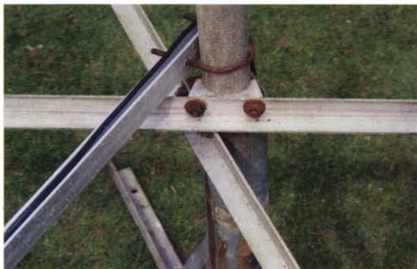
● Fig. 4: Method of fixing the element supports and the coaxial cable support to the mast.
